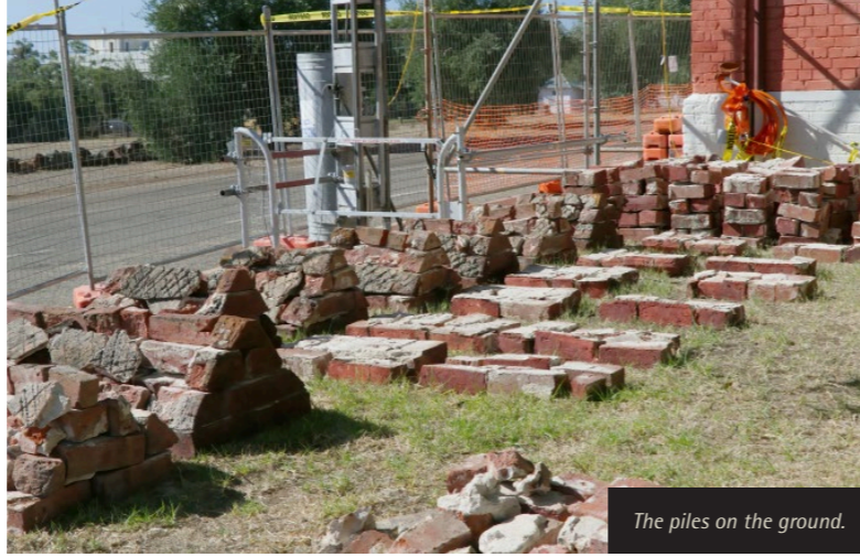
The completed demolition works.
